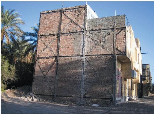
(c) Masonry with Steel Frame (Vulnerability class C).
