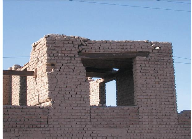
(b) Simple Masonry (Vulnerability class B).
