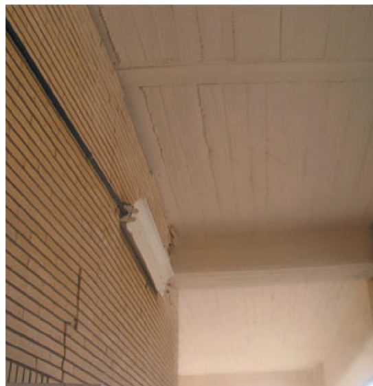
Fig. 28. Out of frame walls parallel to axis 1 between axis C and D, ground floor, with the maximum drift ratio of 0.9%.
