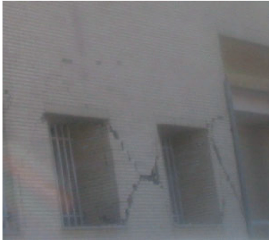
Fig. 24. Failure of the infill wall along the A axis in Fig. 4-b, between axis 6 and 7 in the ground floor, with corresponding maximum drift ratio of 0.9% from the analysis.
