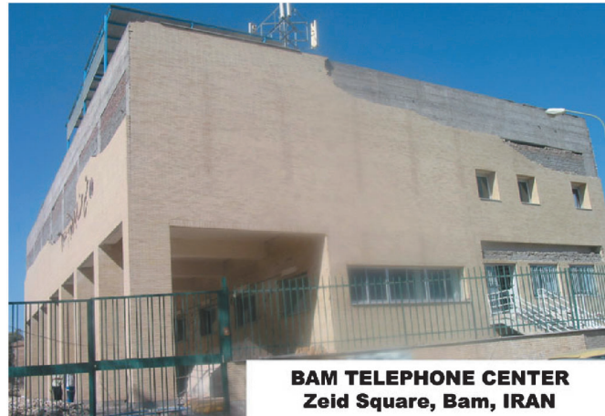
Fig. 1. Bam telephone center RC building after Dec. 2003 Earthquake, South and East sides.
