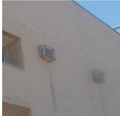
Fig. 25. The infill wall along the A axis in Fig. 4-c, between axis 6 and 7 in the top story, with corresponding maximum drift ratio of 0.1% from the analysis.
