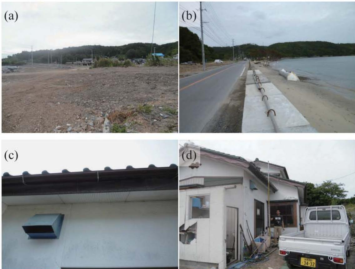
Fig. A228. (a)-(b) Damage at Kugunarihama. (c)-(d) Tsunami trace survey point on a wall of Mr. Sato's house (3.10 m above ground level, M71).
