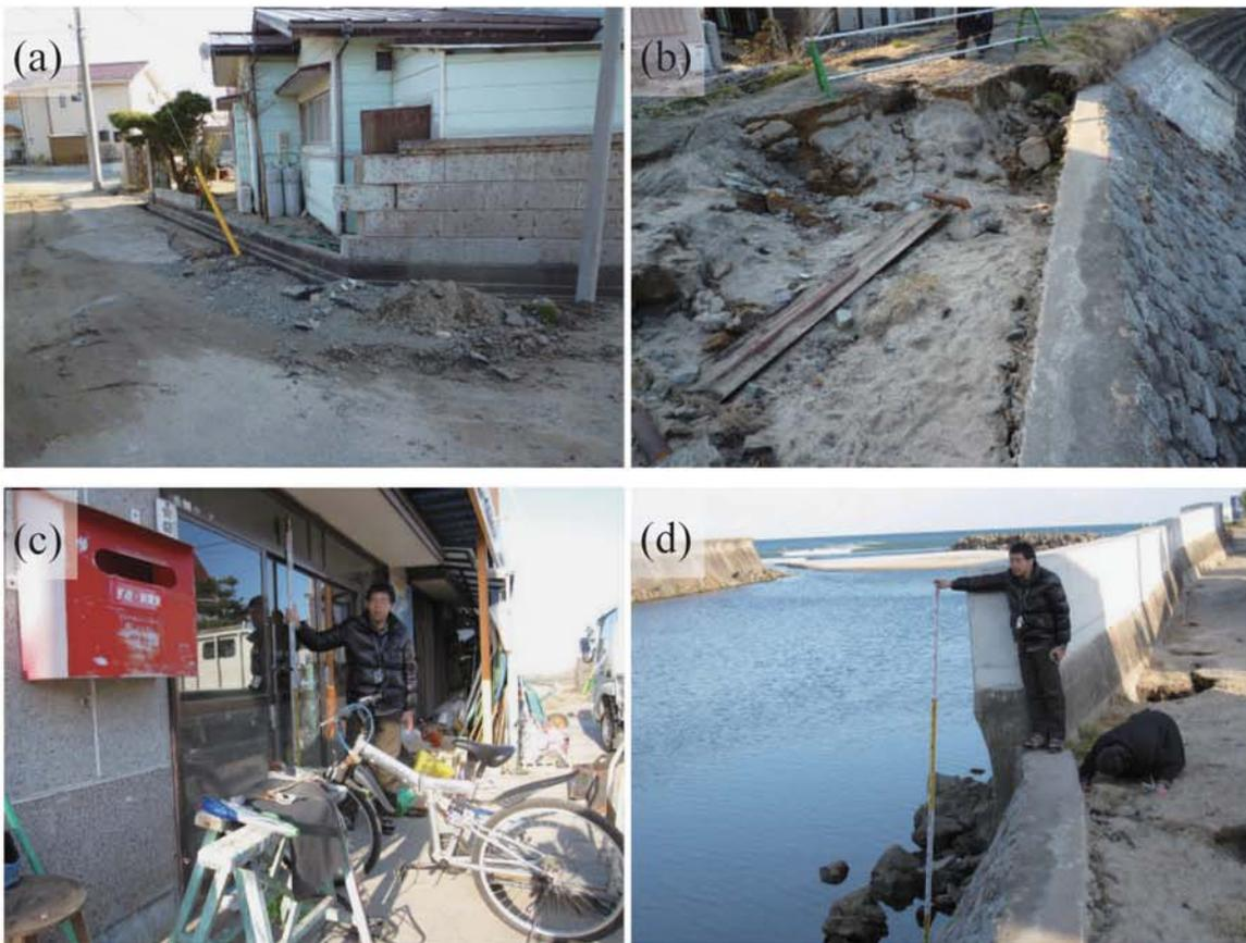
Fig. A252. (a)-(b) Damage at the side of the Sekine River in Hizencho. (c) Watermark on windowpanes of entrance sliding doors of the sign factory Kibokogei at the riverside in Hizencho (0.73m above ground level, B11). (d) Measuring ground height at the survey point based on the water surface in the Sekine River.
