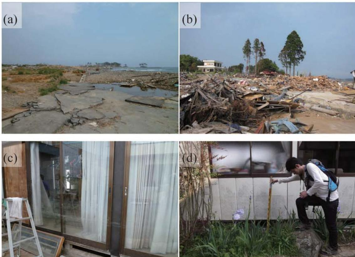
Fig. A144. (a)-(b) Damage at Hajikamisuginoshita. (c)-(d) Tsunami trace survey point on a wall of a house near Hatakeyama ironworks (0.90 m above ground level, M9).
