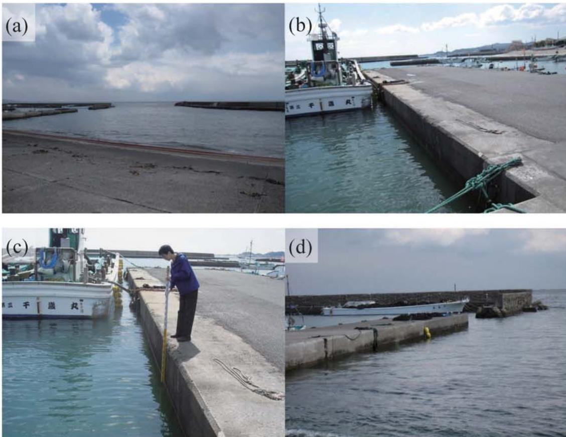
Fig. A344. (a) The Shirako Fishing Port. (b)-(c) Tsunami trace survey point at the top of a quay (C35). (d) The yellow buoys show the upper limit of the Tsunami height at the port (C36).
