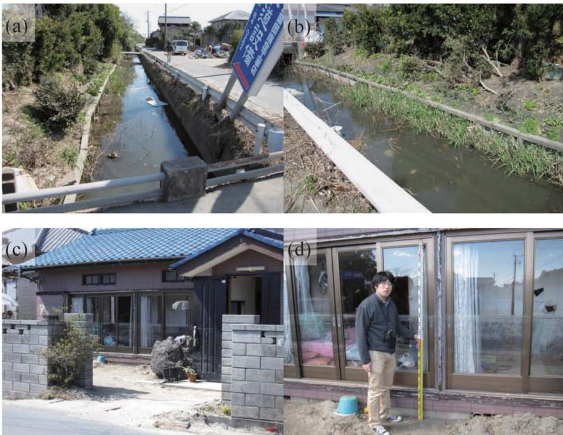
Fig. A312. (a)-(b) Damage due to tsunami run-up through the flume. (c)-(d) Watermark on windowpanes of Mr. Uchida's house (1.27 m above ground level; C14).
