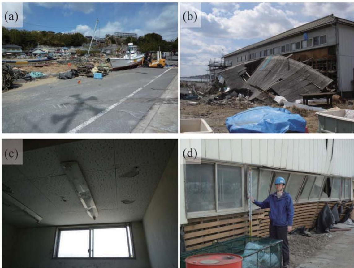
Fig. A266. (a)-(b) Damage at Ose Fishing Port. (c) Tsunami reached the ceiling on the first floor of the fishery association building in Ose Fishing Port. (d) Watermark on windowpanes of warehouse behind the port (1.75 m above ground level, B19).
