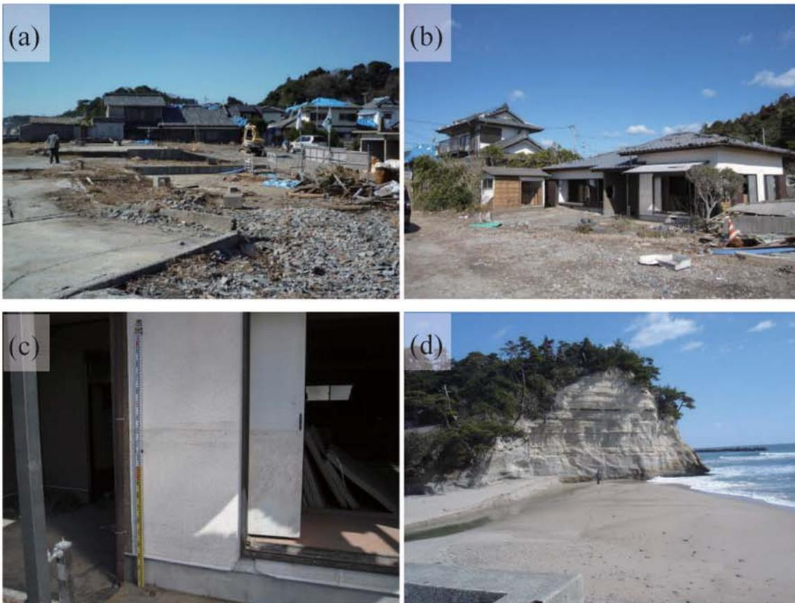
Fig. A260. (a) Damage near the mouth of the Torenzu River in Ogitsucho. (b) Mr. Ikutame's house damaged by tsunami (tsunami trace survey point). (c) Watermark on a wall of Mr. Ikutame's house (1.34 m above ground level, B16). (d) Measuring ground height at the survey point based on water surface in the Torenzu River.
