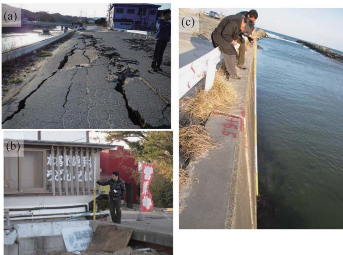
Fig. A254. (a) Liquefaction along the Hananuki River in Arakawa. (b) Tsunami trace survey point at the parking lot of the restaurant Sanukijiyaya (B12). Tsunami inundated the top of the slope at the parking lot. (c) Measuring ground height at the survey point based on the water surface in the Hananuki River.
