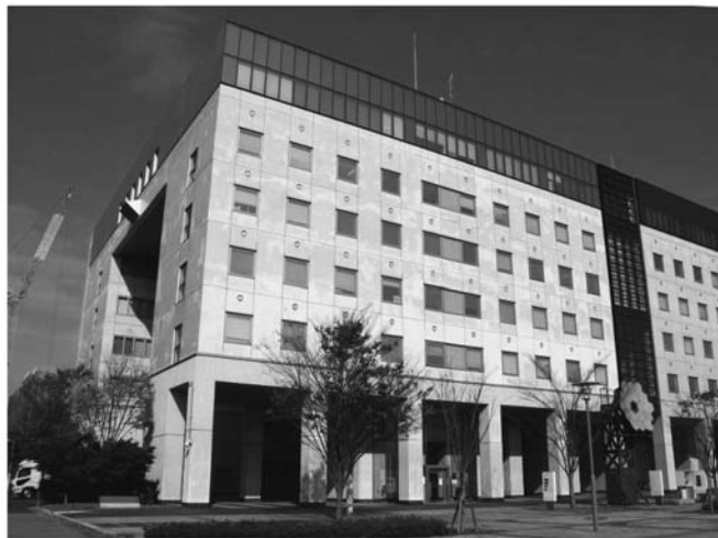
Fig. 7. Plan and Exterior of the Building of Institute for Cosmic Ray Research (“ICRR”) in Kashiwa.
