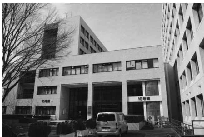
Fig. 10. Joint of Building No. 15 and No. 16.
