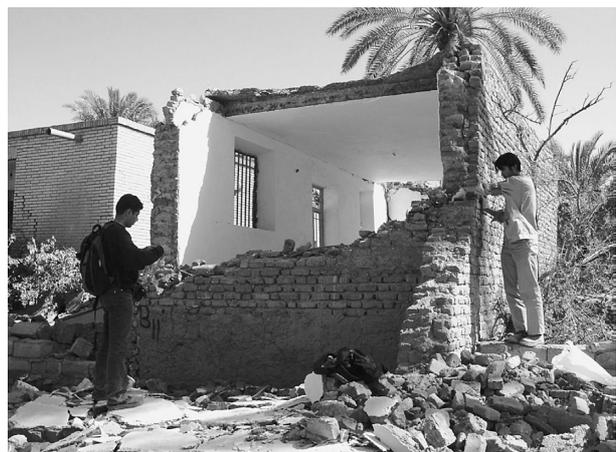
Photo 3. Severe damage to non-reinforced masonry building.
