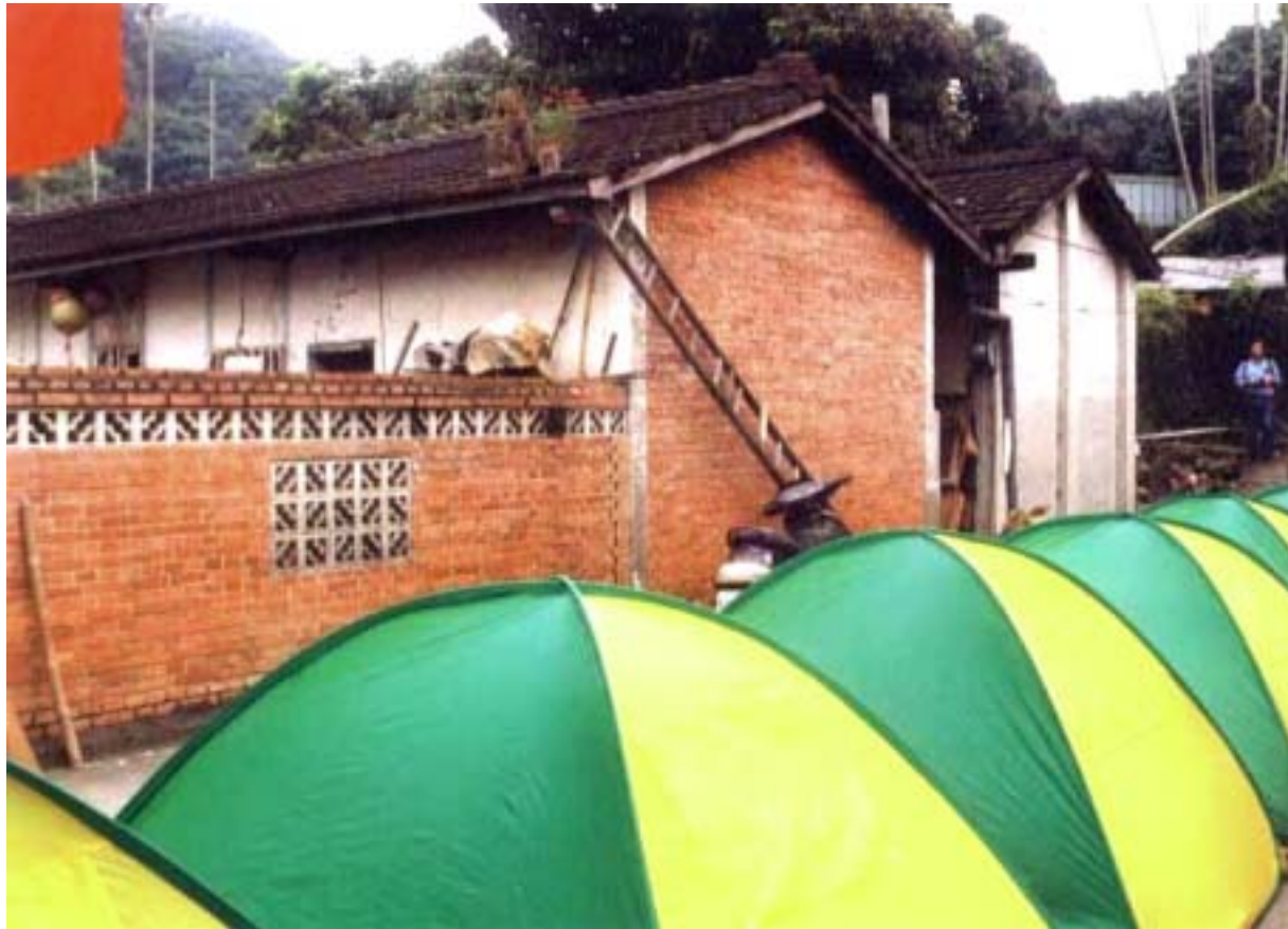
Brick wall close to fault
