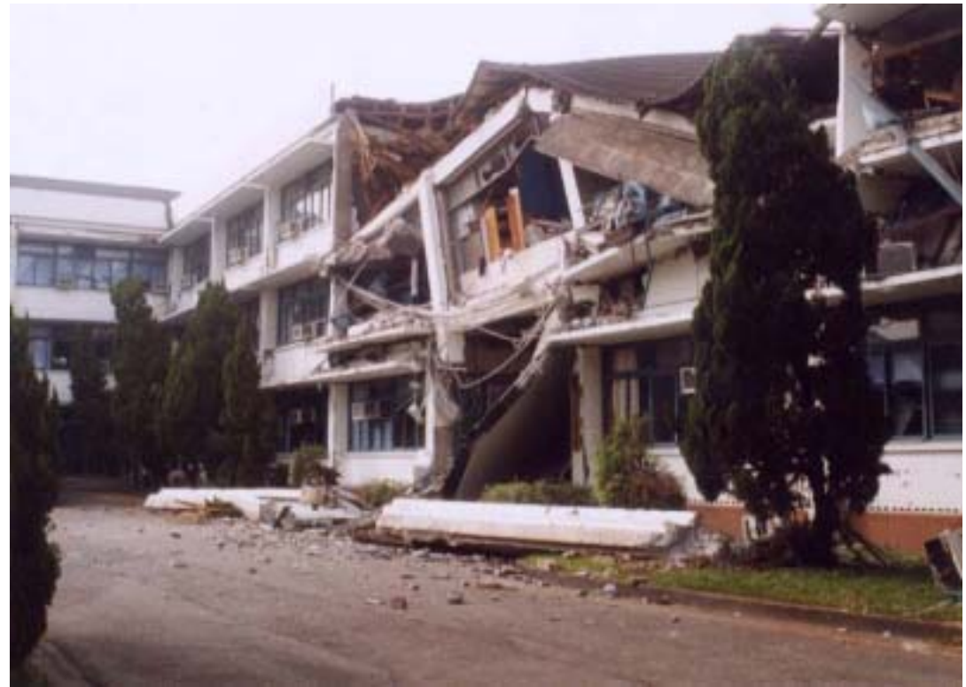
Damaged Government Building
