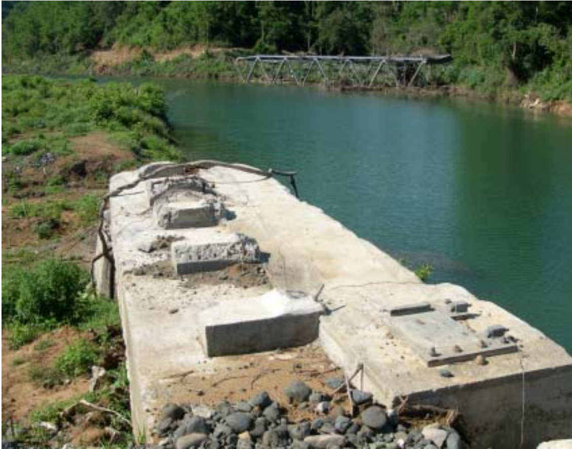
Fig.1 Krueng Sarah truss bridge moved by tsunami (Banda Aceh – Meulaboh, Aceh Besar region)
