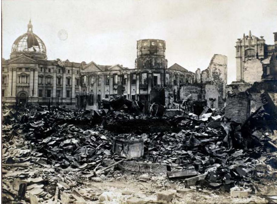
Damage in Yokohama City © Yokohama City Library
