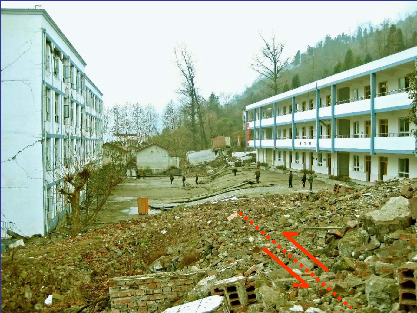
Bailu School in Penzhou City. Surface rupture runs between two classroom buildings with ~3 m vertical offset. No one died.
